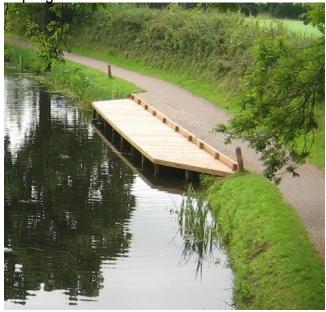
After removing all of the decking it became apparent that some repairs were also needed to the timber frame underneath. These were carried out and the opportunity was also take to create a proper step down from the towpath onto the landing stage, thereby reducing trip hazards and grass cutting maintenance. The Canal Ranger Service and the Tiverton Canal Co are pleased with the work which has also attracted lots of positive comments from visitors.
